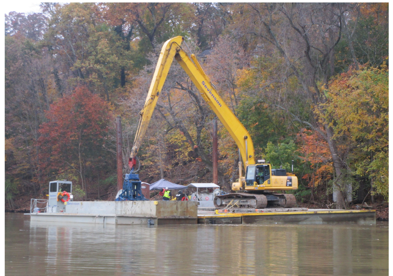
Pompton Lakes Dredging
