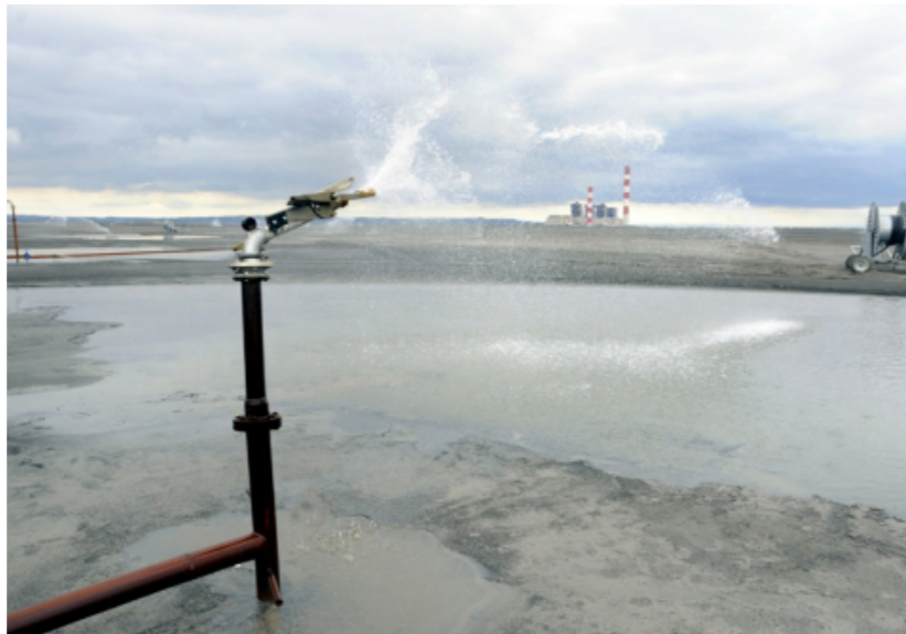
Coal ash pond.
